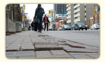
Over time tree roots, traffic and general exposure to the outdoor elements can cause pavers and other hardscapes to shift and become unstable and loose.
