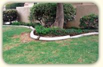
In addition to creating trip hazards, these un-level conditions can cause water to pool, accelerating the deterioration process.
